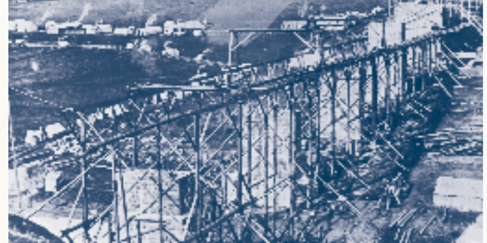
Taradale Viaduct under construction, c1860, black and white photograph from original negative. PROV, VPRS 12800/P1, File H2959
