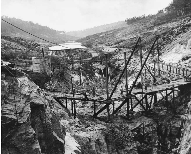
Building the weir wall 1900
