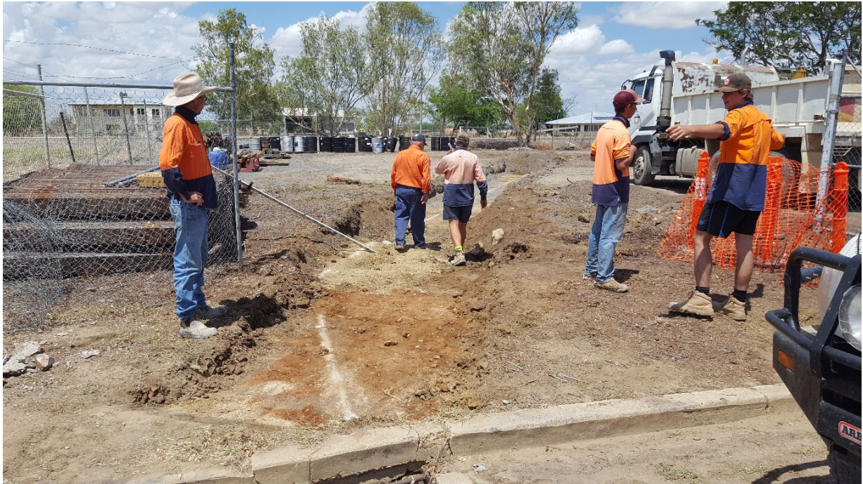
Photo: Exposing the existing concrete pipe at the railway yard.
