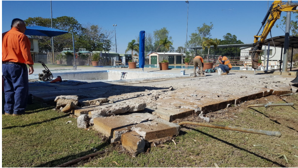
Photo: Demolishing part of the existing slab.
