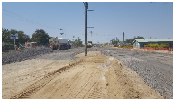
Photo: Carting and placement of gravel pavement.
