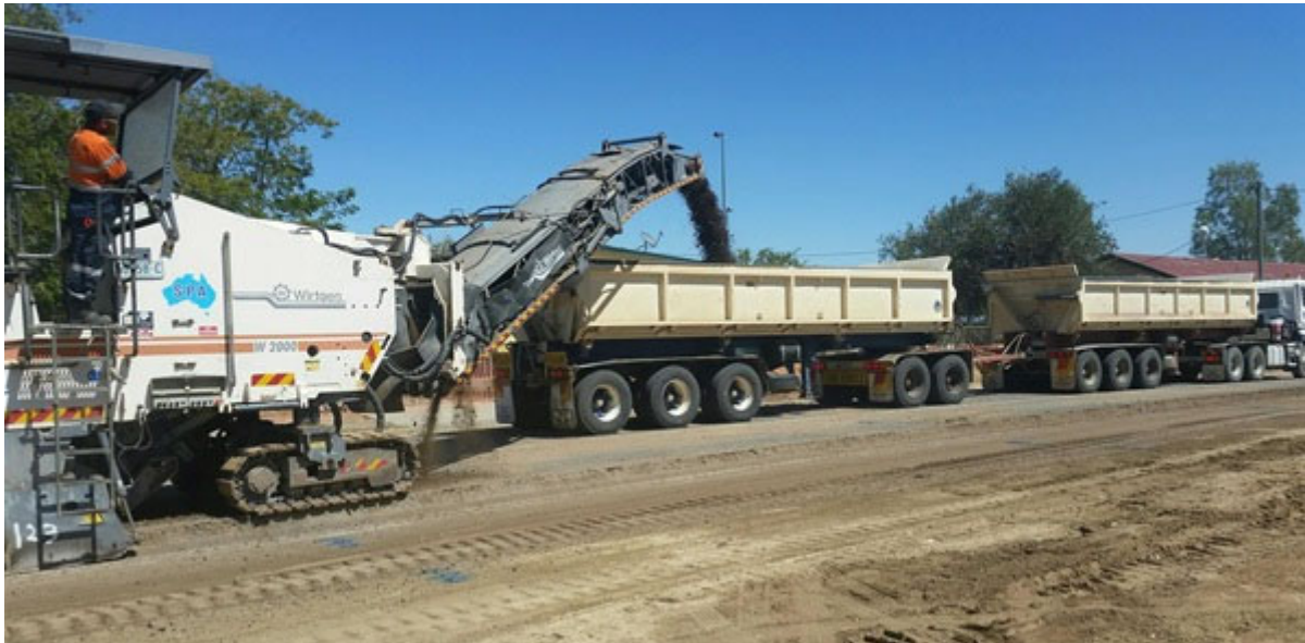
Photo: Milling existing pavement.
