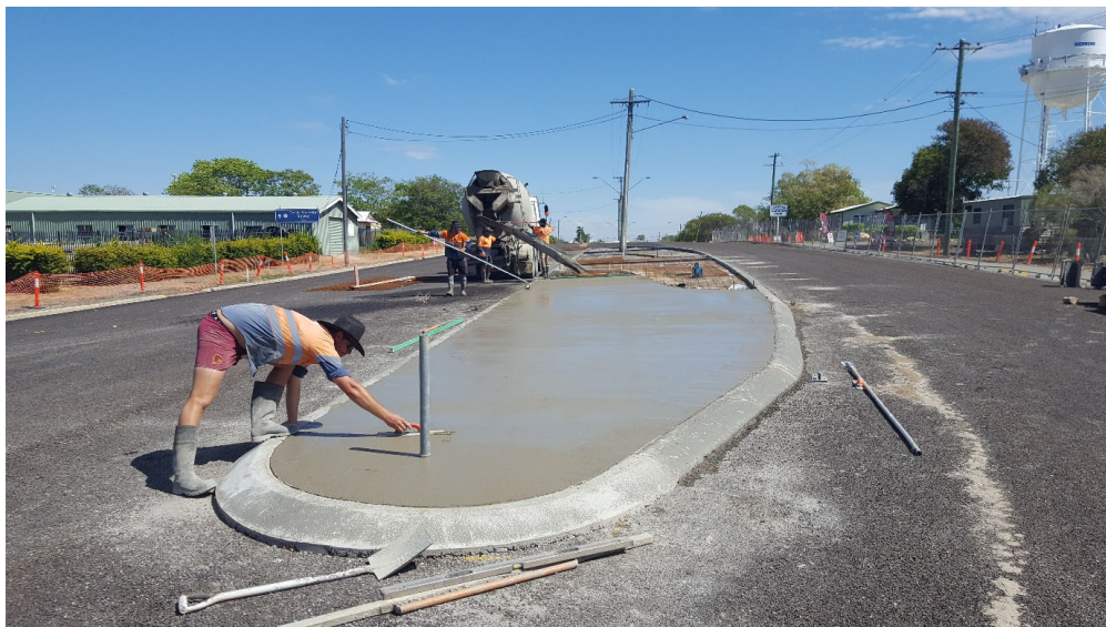
Photo: Constructing Concrete Medians.
