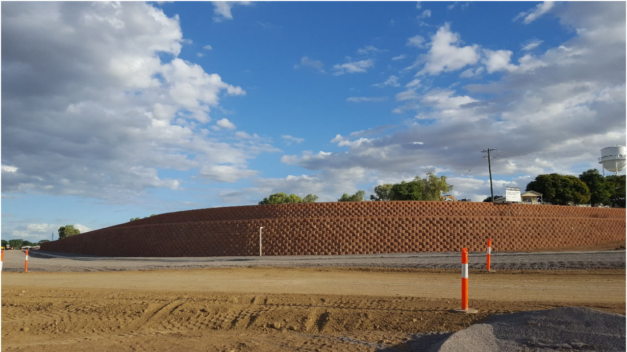
Photo: Completed two tier wall.
