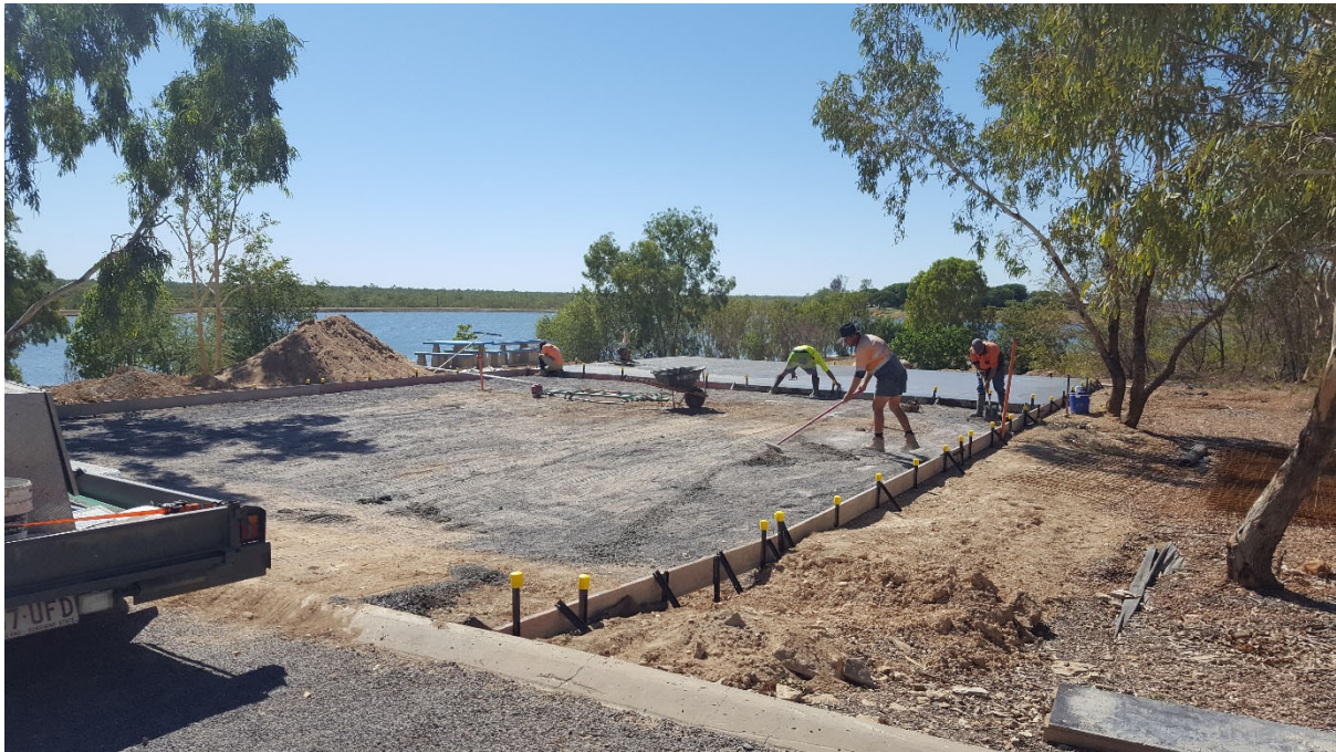
Photo: Construction of concrete slab.
