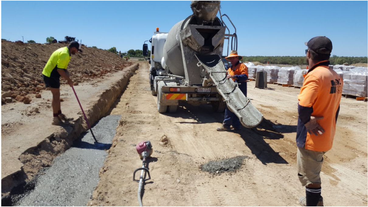
Photo: Pouring footings for the retaining wall.
