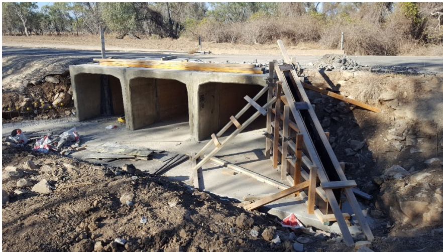
Photo: Widening of culverts at Double Barrel Creek crossing.
