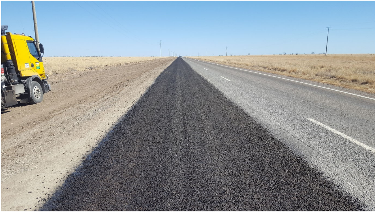
Photo: Sealing patches near Maxwellton.
