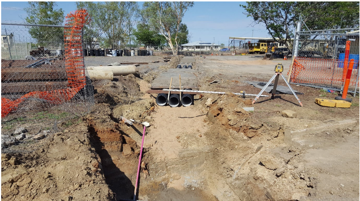
Photo: Replaced with three rows of polyethylene stormwater pipe.
