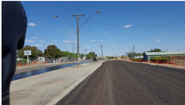
Photo: Sealing works.
