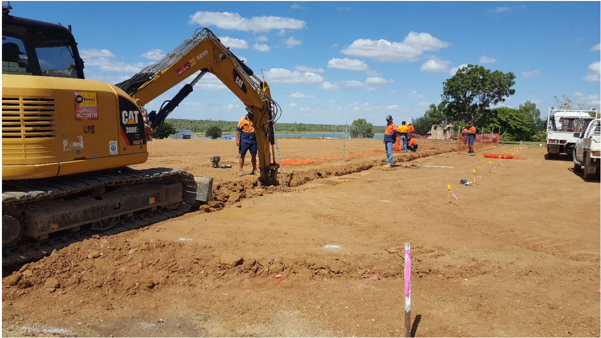
Photo: Installing water supply and grey water drainage to new caravan sites.
