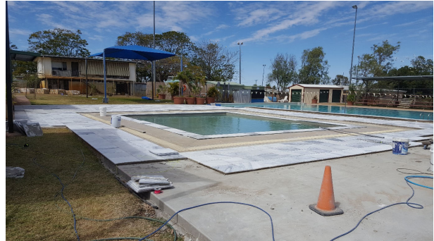
Photo: Stone tiling underway at the wading pool
