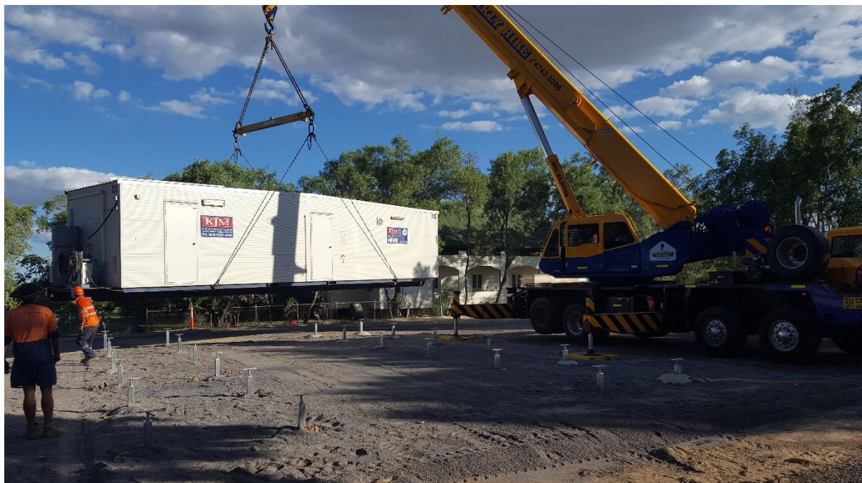
Photo: Installing the ablution dongas.
