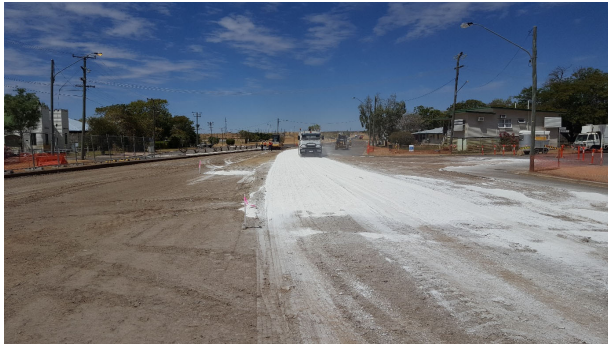
Photo: Lime stabilisation works.
