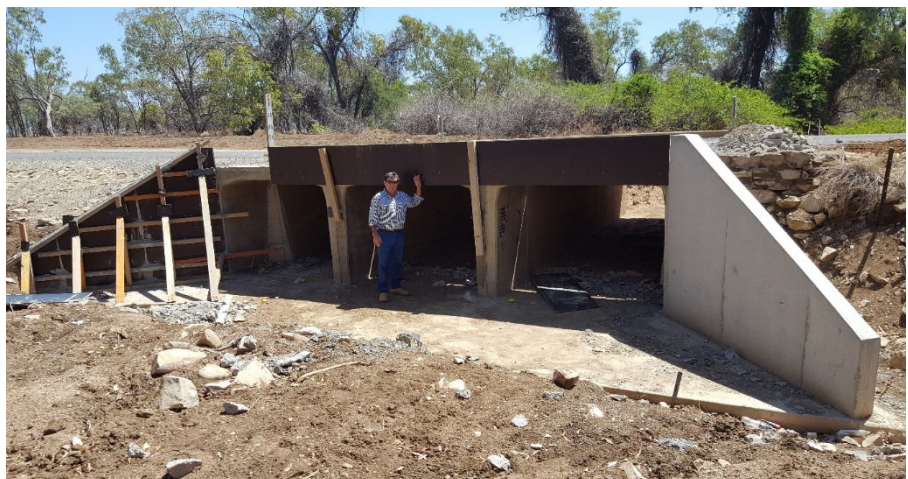
Photo: Widening of culverts at Double Barrel Creek crossing.
