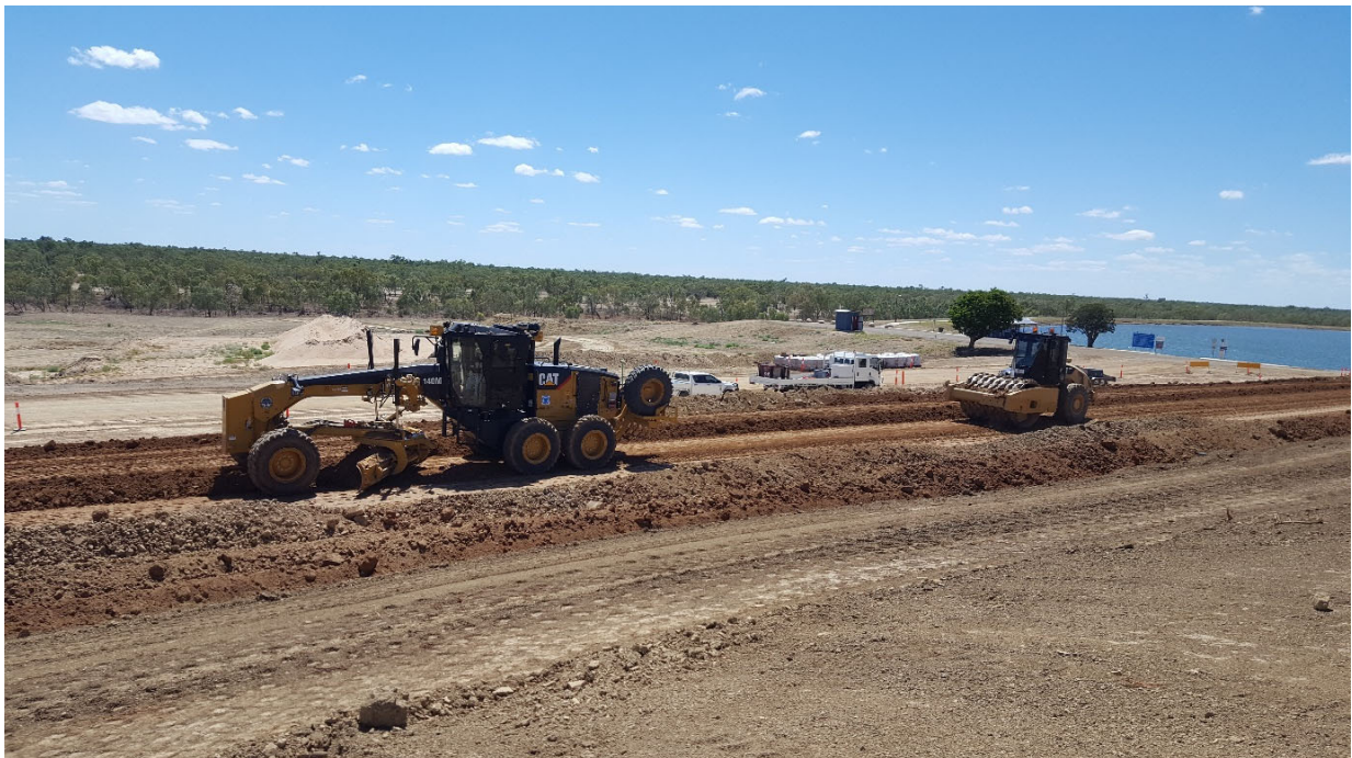
Photo: Placing and compacting fill at the embankment
