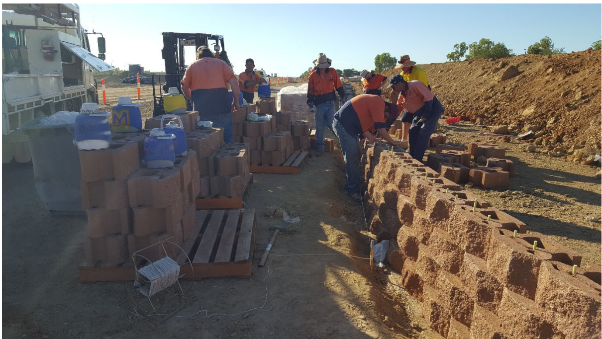
Photo: Placing blockwork.
