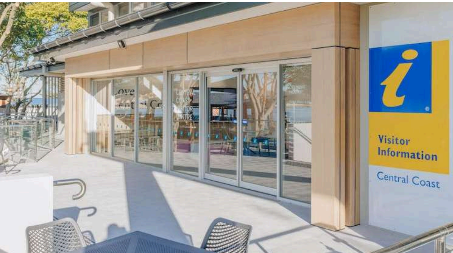
Central Coast Visitor Information Centre, The Entrance NSW. Photo supplied by Isaac Tseng.
